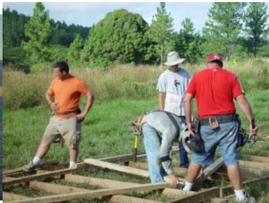
Garrett building trusses.
